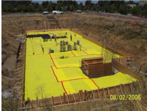
Electrical conduit being installed under the RMI basement slab
