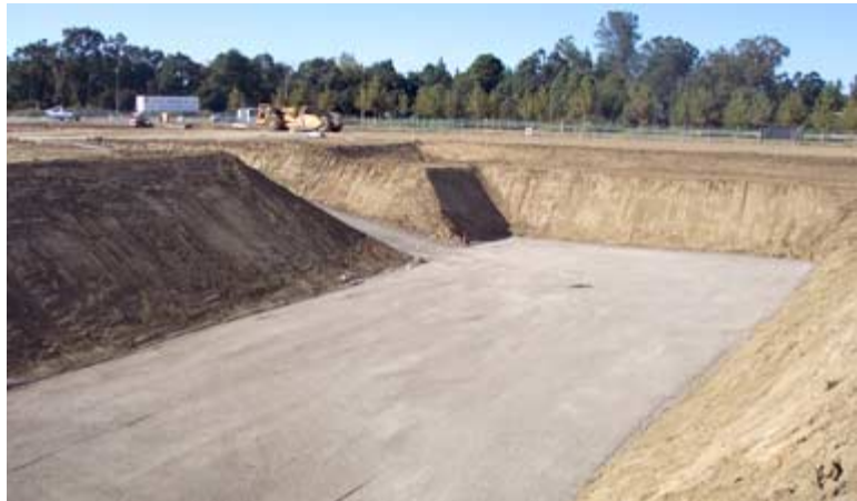
This large hole at the RMI site will remain as the RMI basement, located under the south lab wing
