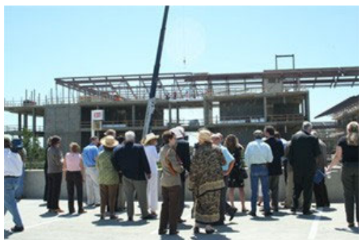
Attendees watch the beam get hoisted into place.
